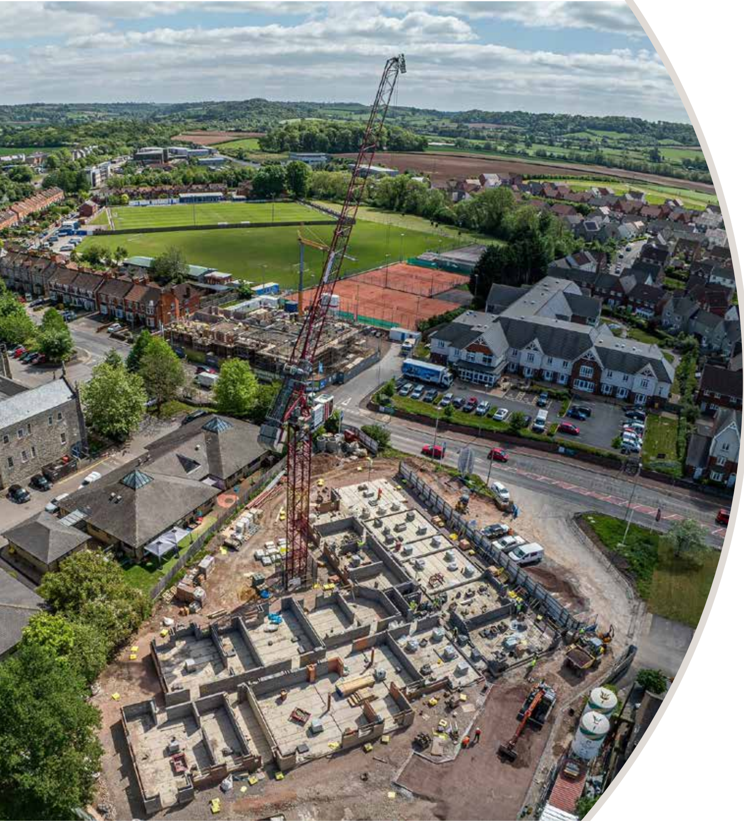
Construction phase at Adam Lock Lodge, Wells
